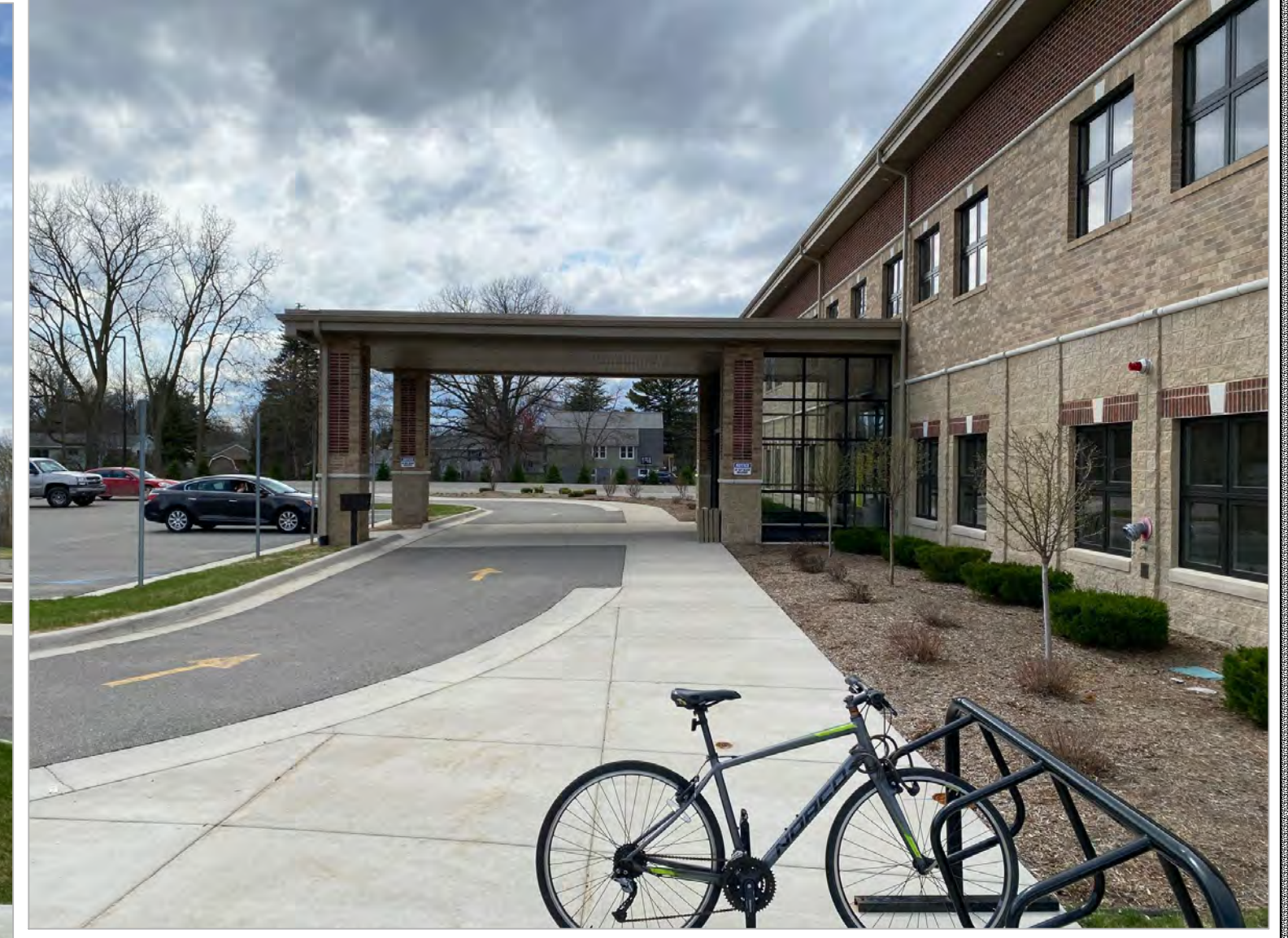
LOOKING WEST AT FRONT FACADE
