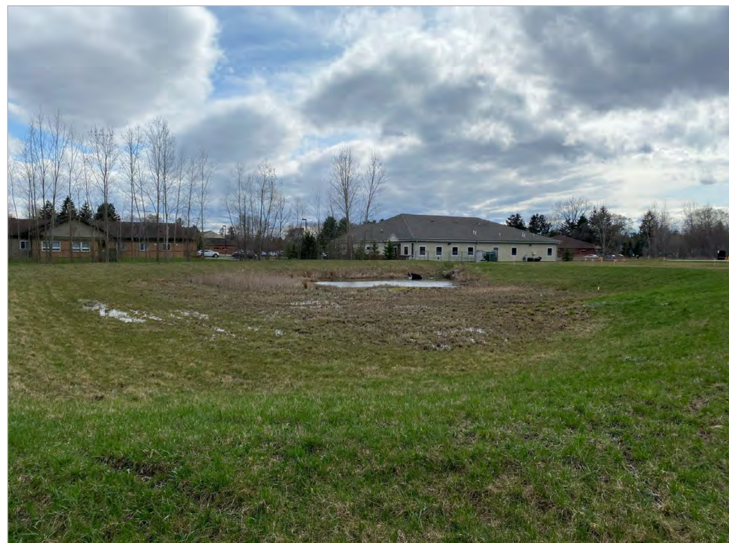
EXISTING DETENTION POND
